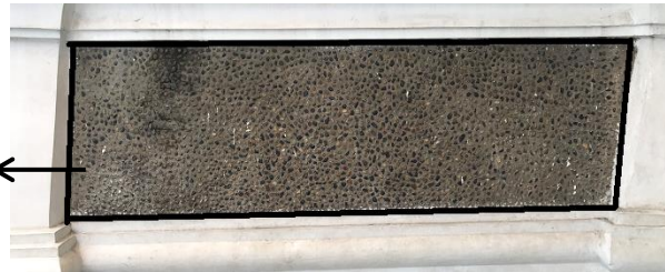
Figure 1b. Mosque wall
