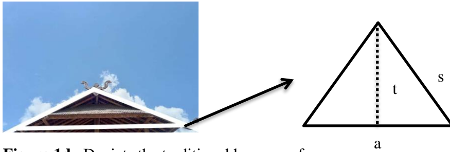
Figure 1d. Depicts the traditional house roof
