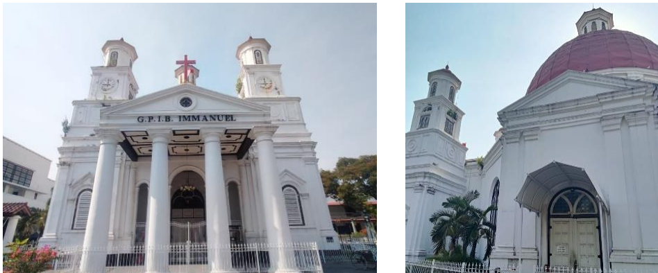
Figure 1. Blenduk church building
